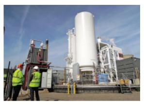
Figure 4: Highview's Liquid Air Energy Storage demonstration plant at Slough. The tank holds 60 tonnes of liquid air. Photo: Highview Power Storage
